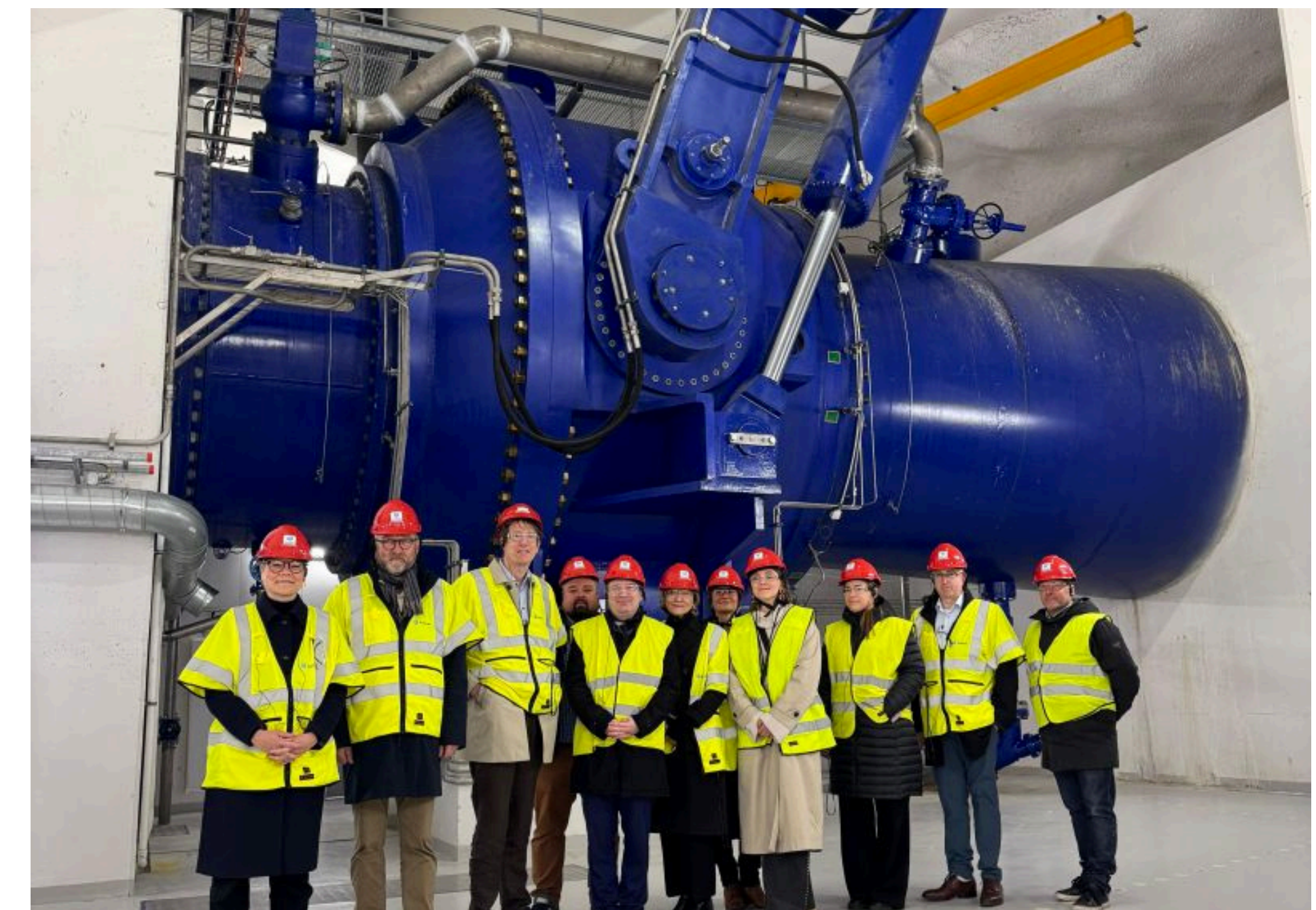
Rana vannkraftverk, a hydroelectric power station.
