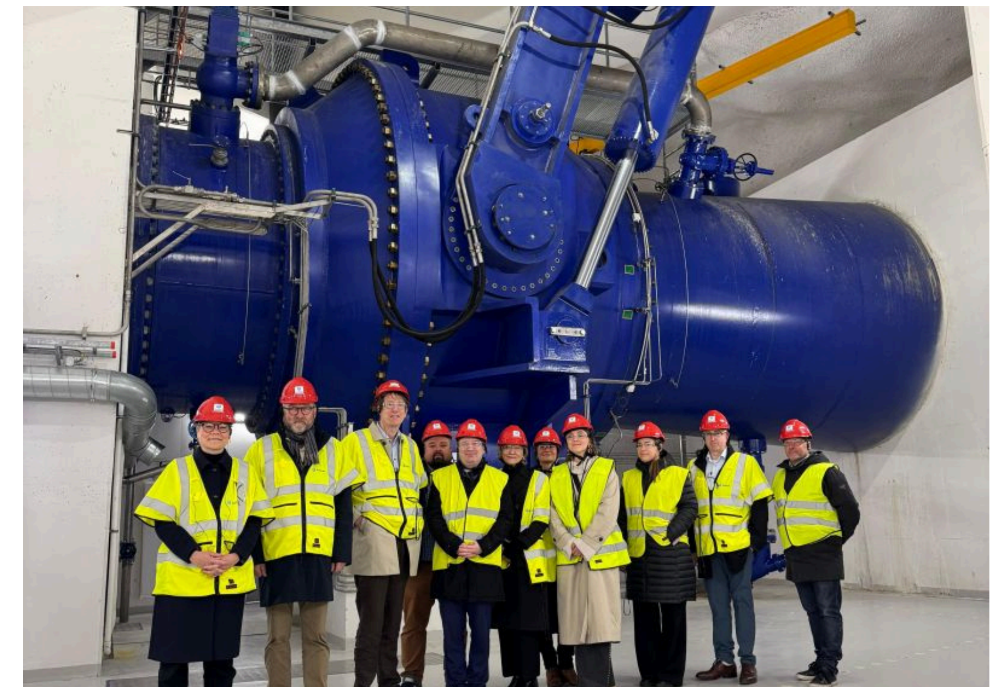
Rana vannkraftverk, a hydroelectric power station.
